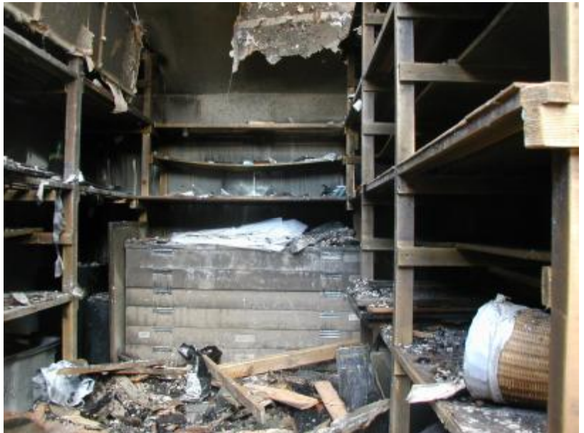
Above. The day after the fire,. The storeroom where all the more valuable items were kept.
